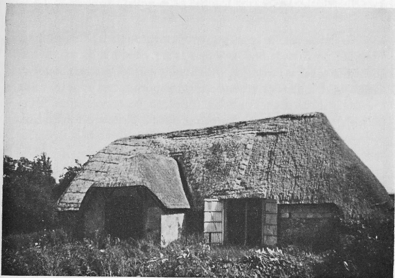
FIG. 1. Barn from north-west.
