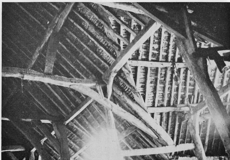
FIG. 4. Interior, truss 3, junction of porch and barn.
